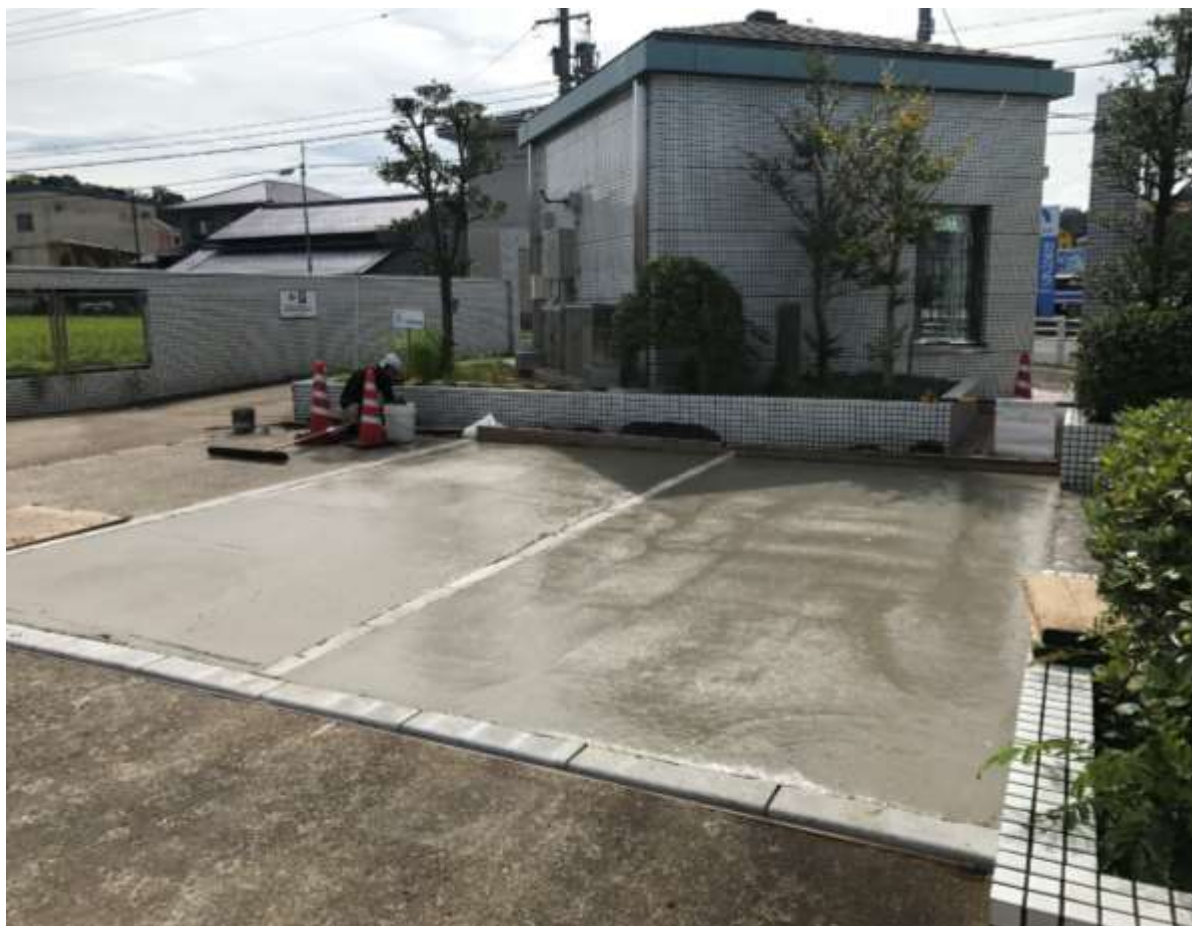
■ After casting concrete
