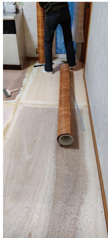
Apply 2.2mm thick Vinyl Flooring Finish layer
