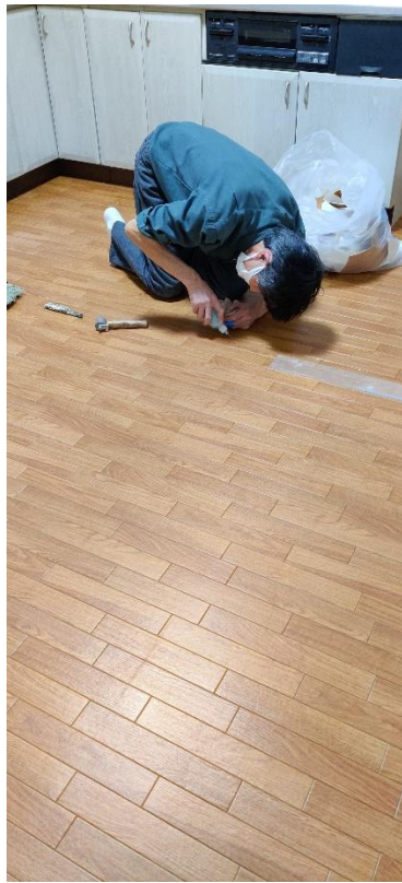
Apply 2.2mm thick Vinyl Flooring Finish layer
